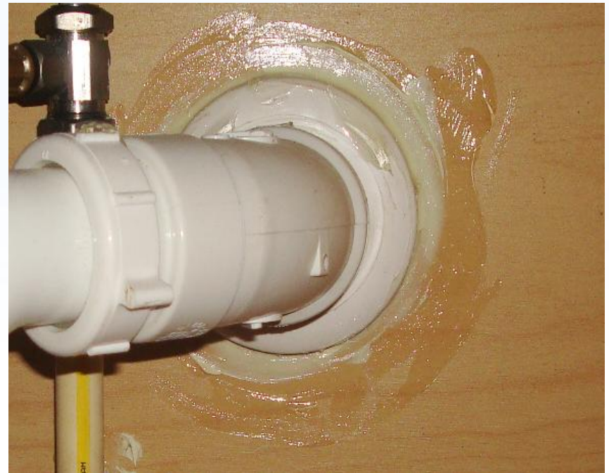
Proper and thorough application
